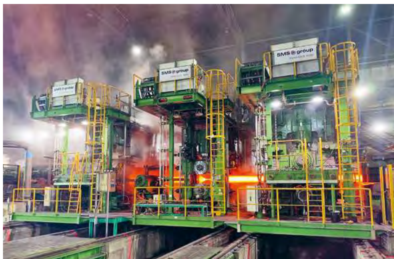
CCS 1500 universal stands at Nucor Yamato Steel after the revamp of rolling mill no. 1 in Blytheville, USA
